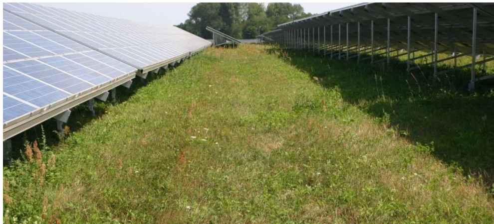
Figure 1-5: Row spacing of approx. 5.5 meters in the Finow II solar farm (Brandenburg). Area exposed to sunlight approx. 4 - 4.5 m wide
