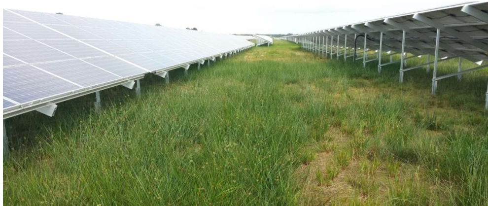
Figure 1-5: Row spacing of approx. 5.5 meters in the Finow II solar farm (Brandenburg). Area exposed to sunlight approx. 4 - 4.5 m wide
