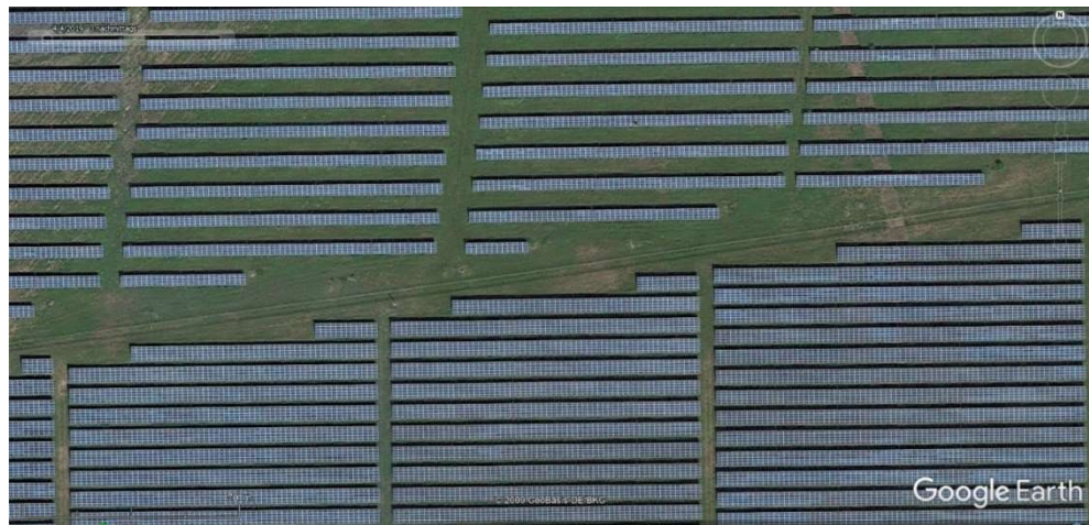
Figure 1-9: Comparison of different design methods using the example of 2 solar parks on the former Fürstenwalde airfield (Brandenburg). Aerial photo source: Google Earth ©2019 GeoBasis-DE/BKG ©2009, date taken 06.06.2018, modified, orientation north
