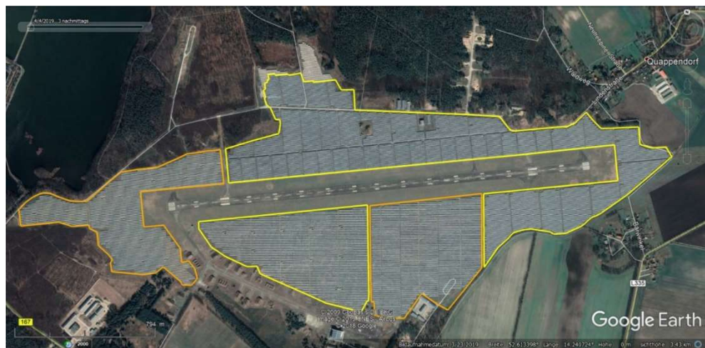
Figure 1-7. The other 3 photovoltaic facilities have wider row spacing.
